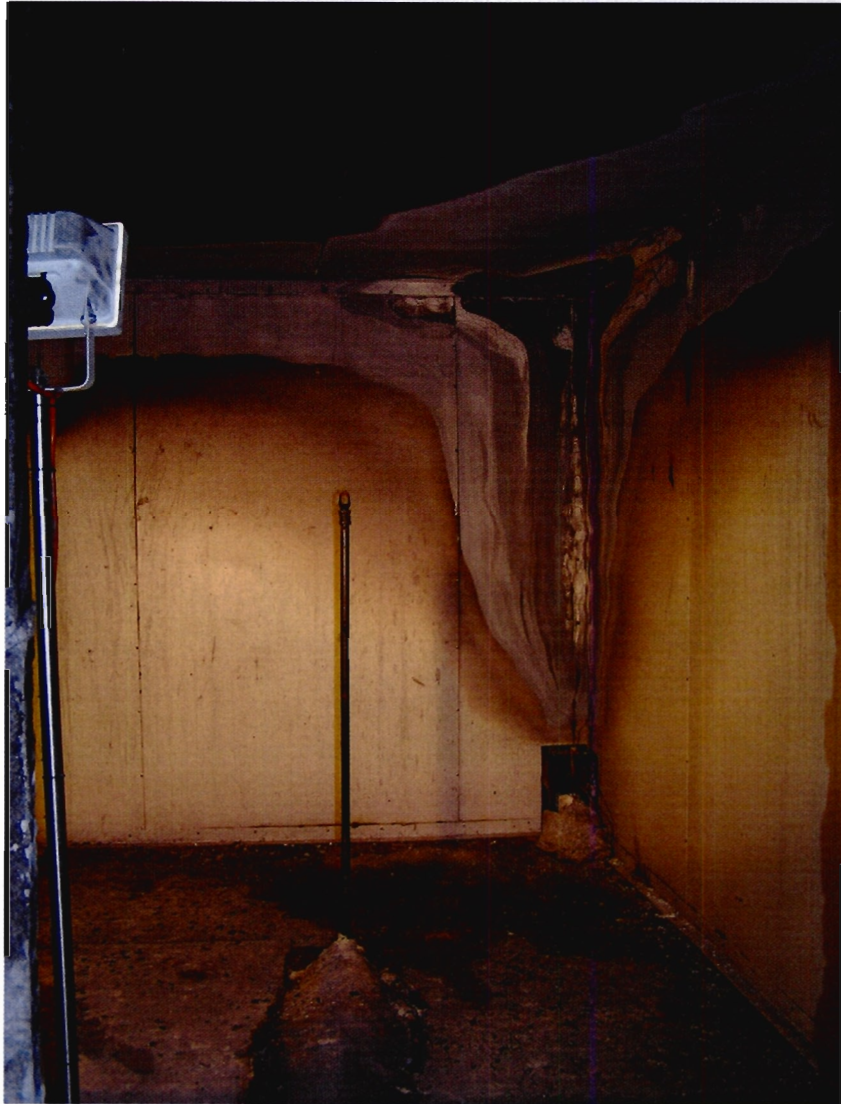
Figure 9: Specimen after fire exposure
